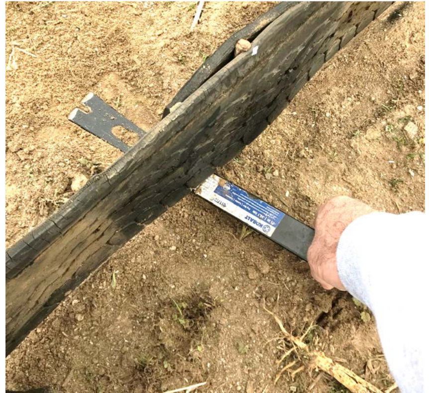
Pry bar used to reposition lumber on stake.
