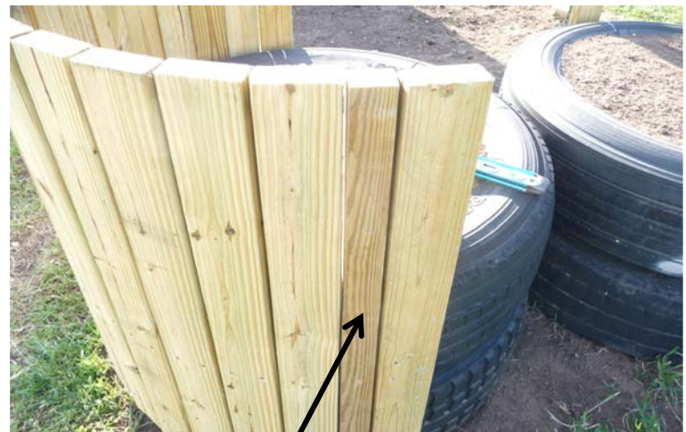
Custom cut frame member
