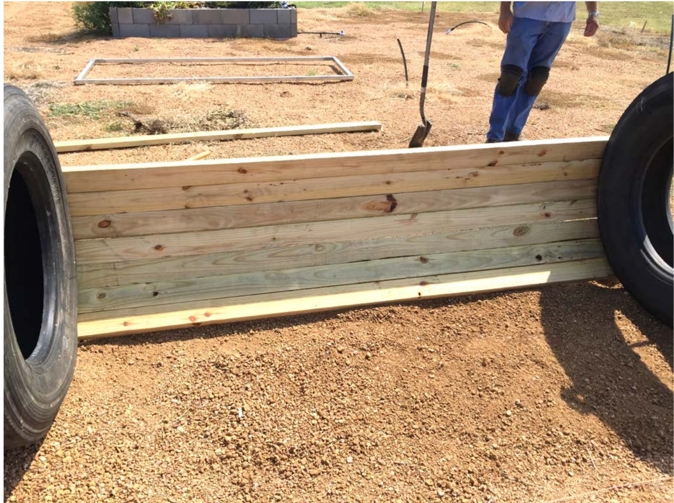
One side of planter installed.
