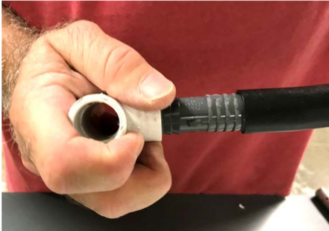
Inserting free end of coupler into poly pipe.
