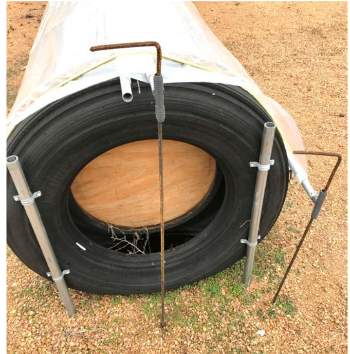
Reels locked in place using rebar stakes.
