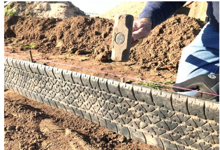
Rubber Lumber Bed under construction
